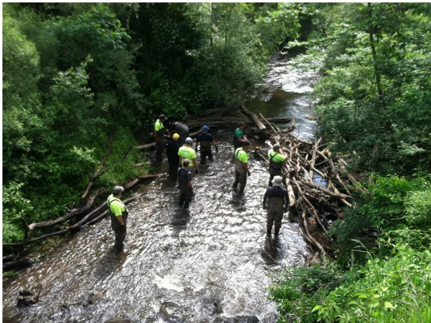
Large woody debris cleanup looking downstream from Clarkson Road bridge.
